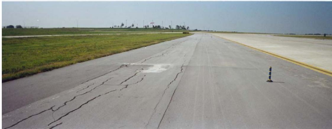
Sulfate-Induced Heave “Speed Bumps” in Lime-Stabilized Subgrade
